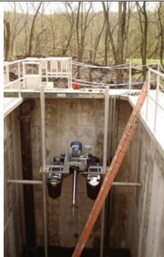
This pre-start up photo shows how the unit is able to ride vertically up and down on stainless steel slide-pole assemblies as water levels in the tank change.
