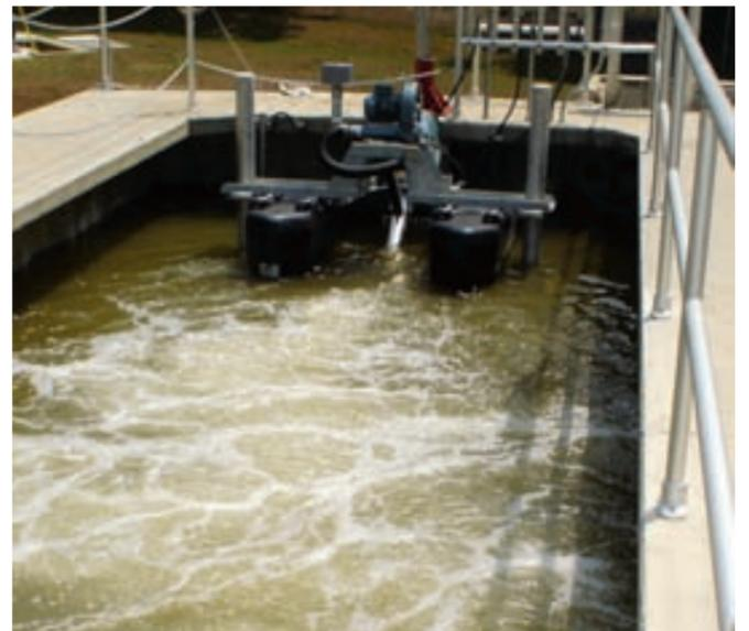
The Triton dual-function aerator/mixer provides process flexibility to nitrify and denitrify as well as facilitate biological phosphorus removal by changing controls to allow for anoxic mixing steps during the cycles.
