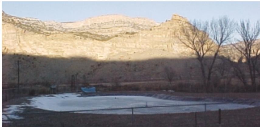
lagoon and wetland system since evapotranspiration rate and biological degradation rate are lower in the winter and higher in the summer. In addition, the lagoon/wetland system can easily accommodate organic and flow variations by mixing influent in the lagoon and providing significant storage in the wetland basins. Wetlands with cattails and rushes are able to tolerate water level and pollutant concentration fluctuations.
