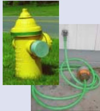
Attach an HPR to the hydrant that is closest to the customer's building and on the same main.
