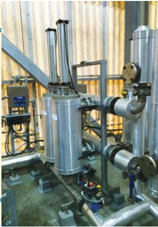
A mechanically cleaned filter recovers titanium particles and protects Global Titanium's ultra filter.
