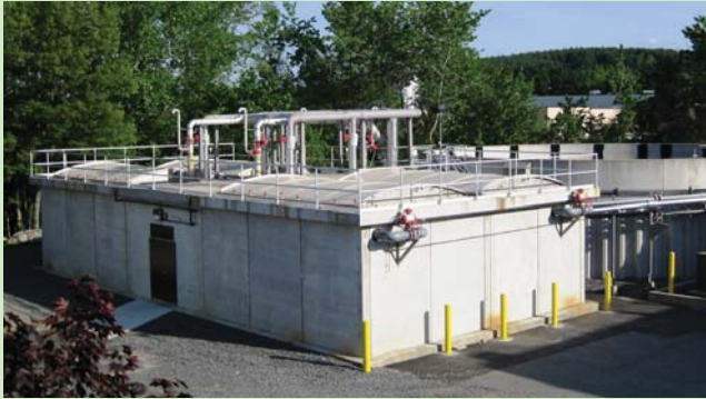
Ken's Foods leveraged an anaerobic membrane bioreactor.
