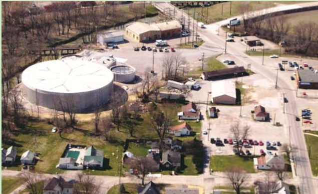
Bellisio Foods selected a system that allows it to meet its discharge limits.
