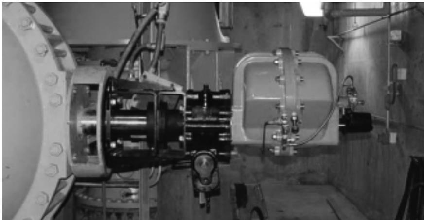
*This 48" ball valve with actuator includes a fabricated linkage kit to the valve.*
