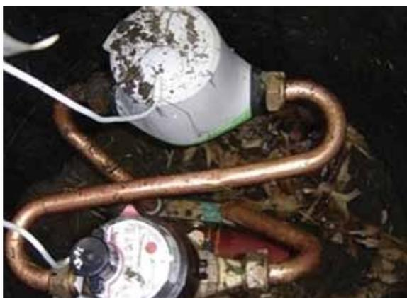
As part of a research study at 23 residences, a static meter (top) sits next to a mechanical meter (bottom) in a tandem setting to measure and compare water usage rates between the two meter types.
