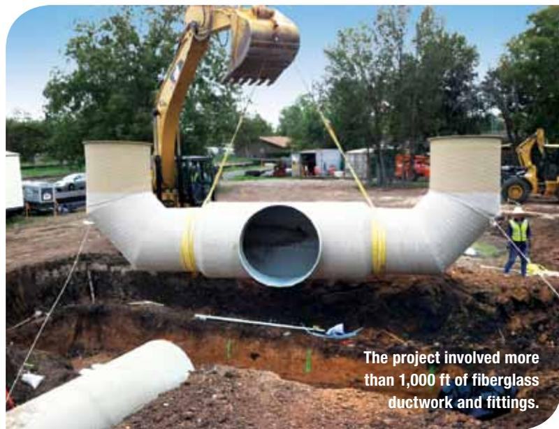
The project involved more than 1,000 ft of fiberglass ductwork and fittings.
