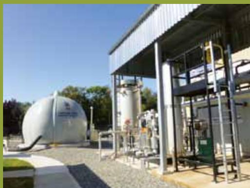
Excess methane gas from anaerobic digesters is collected and converted into usable electricity in a new biogas engine.
