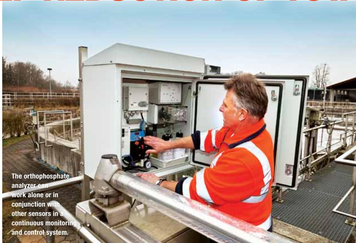
The orthophosphate analyzer can work alone or in conjunction with other sensors in a continuous monitoring and control system.
