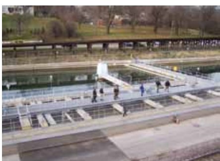
Completed flocculator/sedimentation basins.
