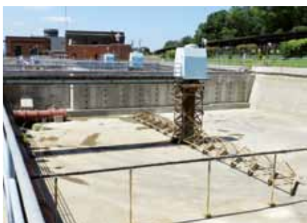
A view of the sedimentation basin as the project nears completion.
