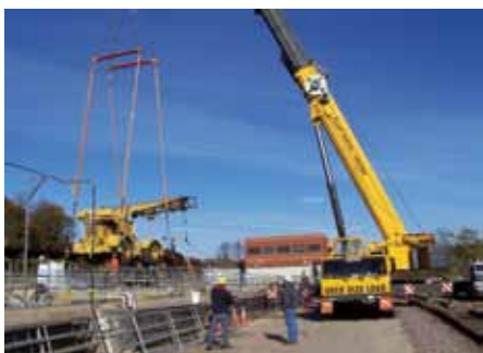
A crane is lowered into one of the existing flocculation basins.
