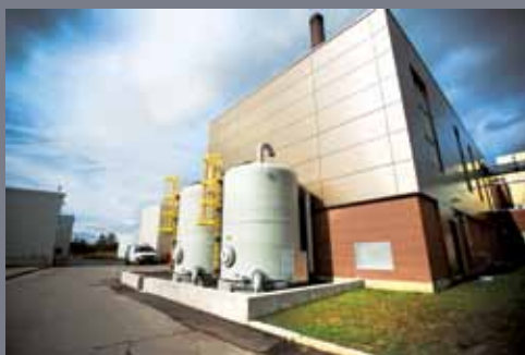
In addition to being a fully operational wastewater treatment plant, the Greenway plant also functions as a demonstration facility for technology testing.
