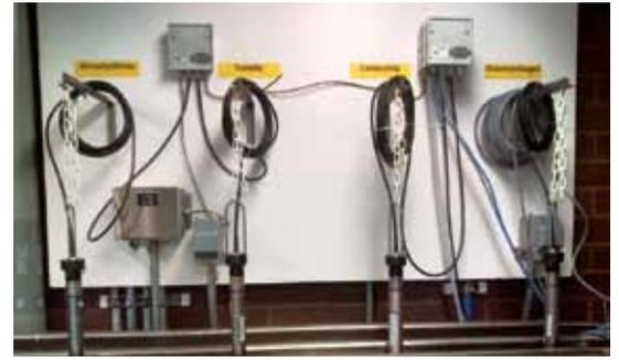
The most common target for aeration system optimization is DO concentration. The options for DO control range from simple manual adjustments based on measurements from grab samples to automated adjustment of blowers and valves with online measurements.
