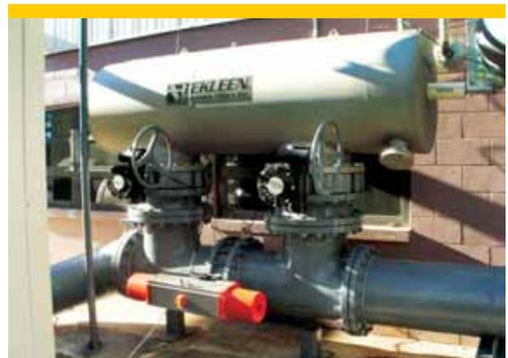
The filters eliminate the need to clean the strainers, allowing the equipment to stay online.
