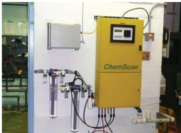
The ChemScan UV-2150S chloramination analyzer monitors all four key parameters from two sample points.
