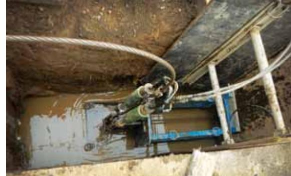
Static pipe bursting was the best way to complete the project with the least disturbance to the surrounding area.
