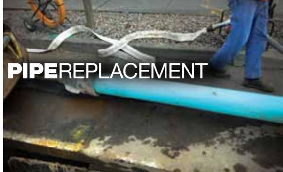
Clean Water Services decided to replace an aging portion of concrete sanitary sewer main in Beaverton, Ore., that was experiencing excessive tree root infiltration.
