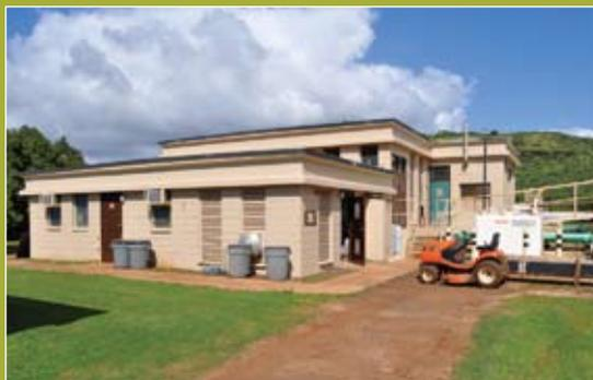
The plant will be upgraded to 700,000-gpd capacity and will include a process train that discharges R-1 quality effluent.
