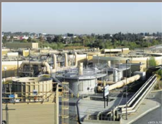
LACSD recently invested $23 million in collecting, transporting and treating foul air from JWPCP's solids processing areas.
