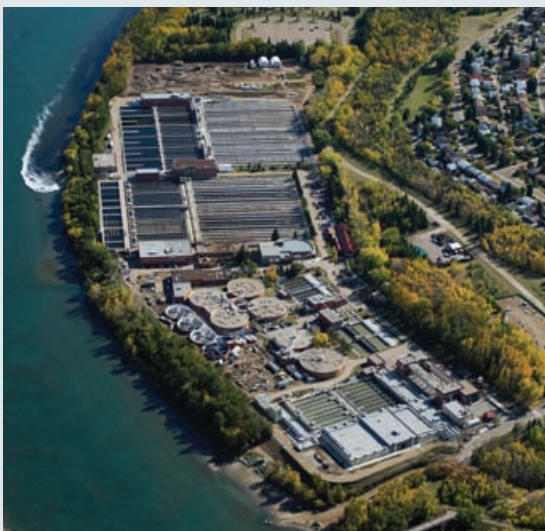
Natural treatment, biogas conversion and water reuse are among Gold Bar WWTP's ongoing areas of focus.
