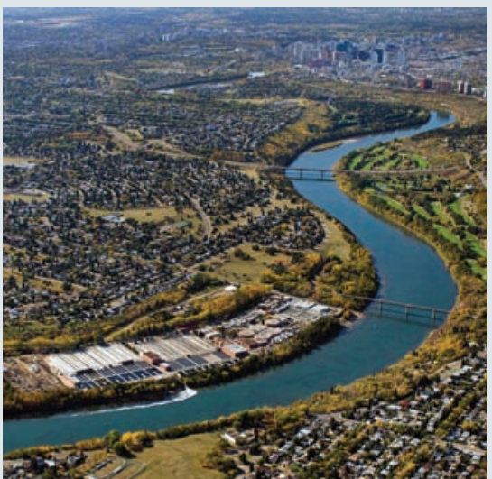
The WWTP is situated along the North Saskatchewan River and discharges treated water into it.
