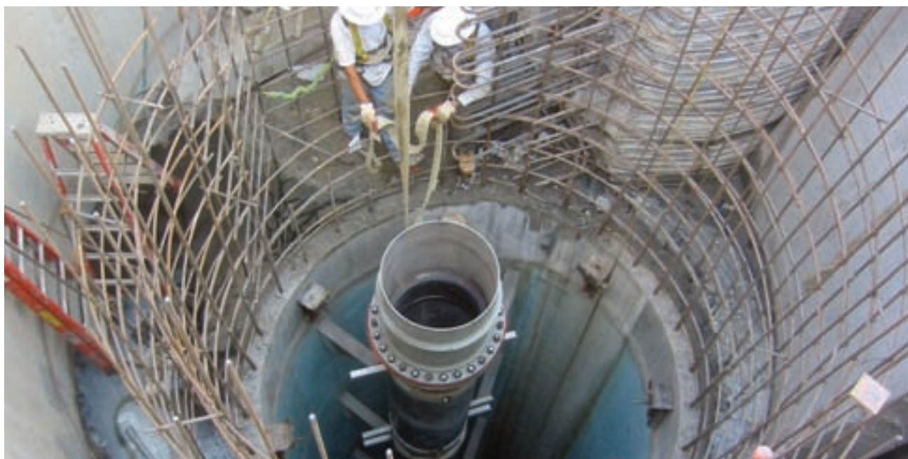
An overview of Charleston's water system sewer tunnel replacement program
