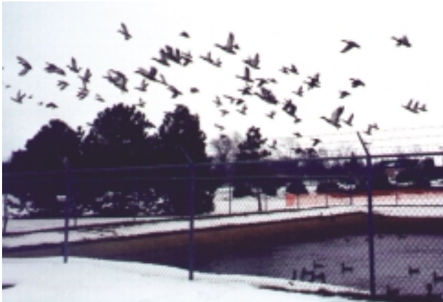
The settling basin for filter backwash water at Morton accumulates iron sludge and provides a habitat for ducks.
